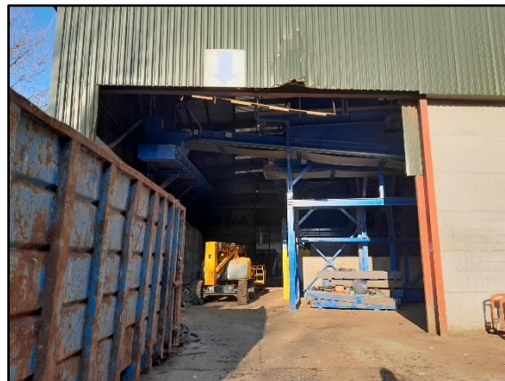
Location of new rapid close door
